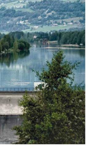
two reservoirs to profit from price fluctuations on the electricity market. In times of low demand or high production, when power is cheap, water is pumped into the higher reservoir. During times of peak demand the water flows back down through the turbines, generating power that is then sold at peak prices.
